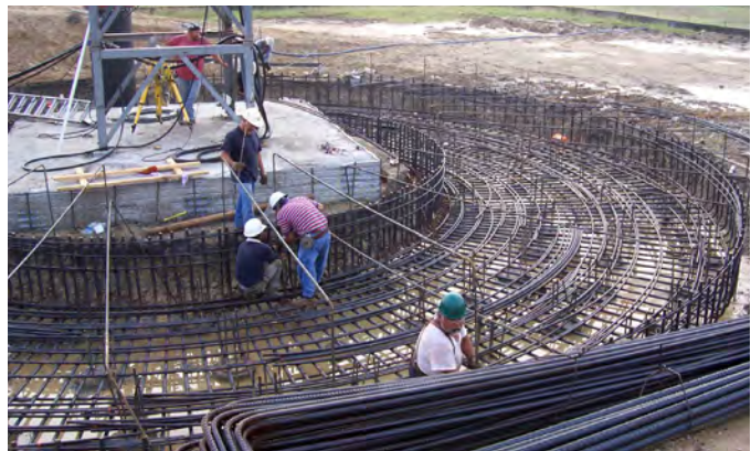
Rebar for pile cap
