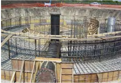
Foundation rebar and piping
