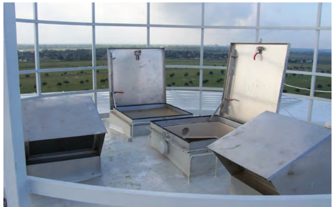
Tank roof with hatches, vents, and rail
