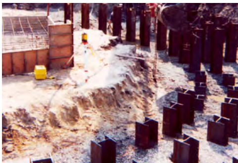
Driven steel piles
