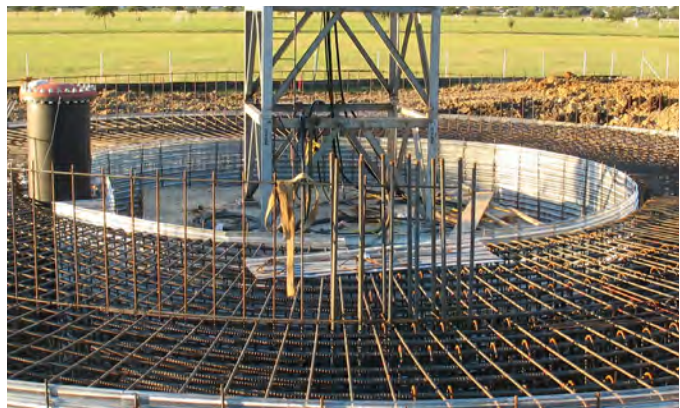
Rebar for pile cap
