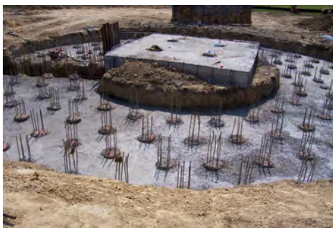
Concrete piles
