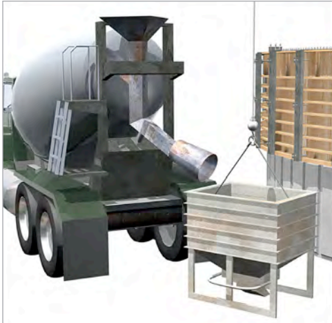
One truckload per form segment
